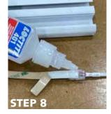
Put a small drop of instant glue on the back of the connector.
